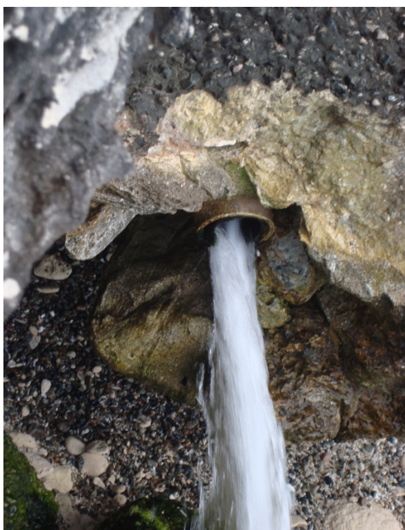
Figure C11 Pipe for discharging brine (hypersaline water) from desalination plant at Fays Bay, photograph by C. Loos
