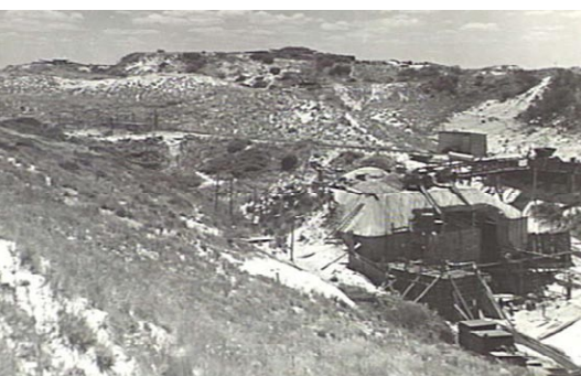
plotting rooms under construction, 1942 [3]
